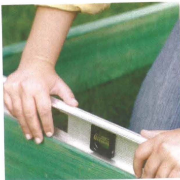
4 Check positioning of frame with level. Adjust height with shims if needed. Secure frame to ground with raised bed stakes (included in corner bracket kit), then cover with plastic caps (also included in kit).
