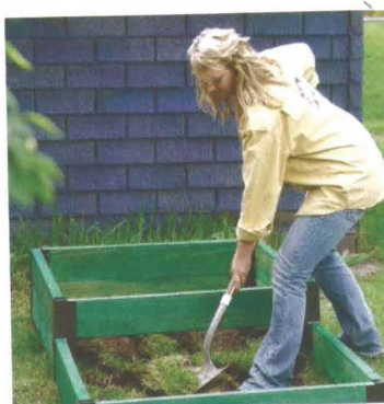
5 Excavate sod beneath the frame to a depth of 6 inches to free up space for root growth. Remove sod from shallower front tier; simply turn sod over in the deeper tier in back.
